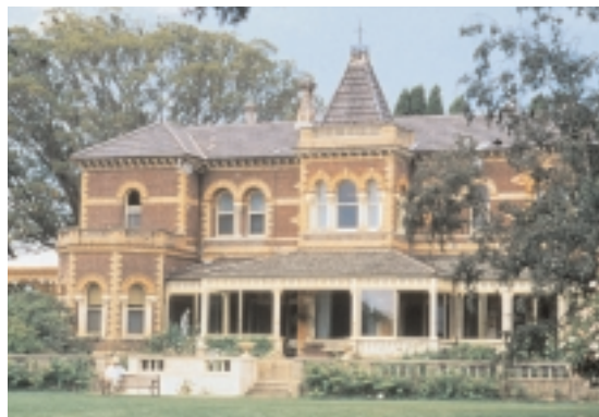
Rippon Lea, a prominent example of early Melbourne polychromatic brickwork, designed by Joseph Reed. Photograph courtesy National Trust (New South Wales).
